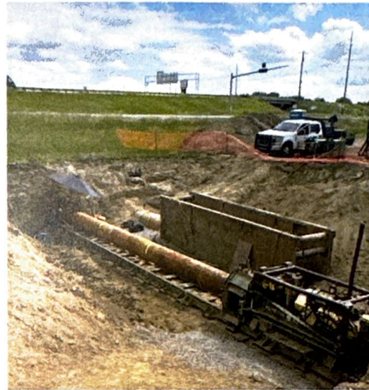
Left photo: 6/4/25, crew working on the new 12" sewer main near MH-10 Right photo: 6/12/25, second 24" bore under the I-90
